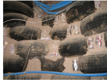
Earthship wall construction
